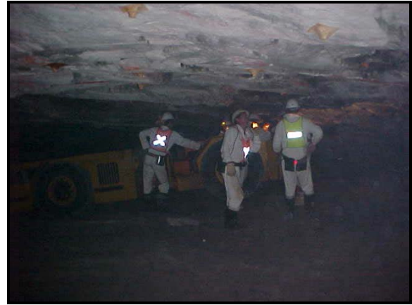
General view showing mining height and hanging wall conditions
