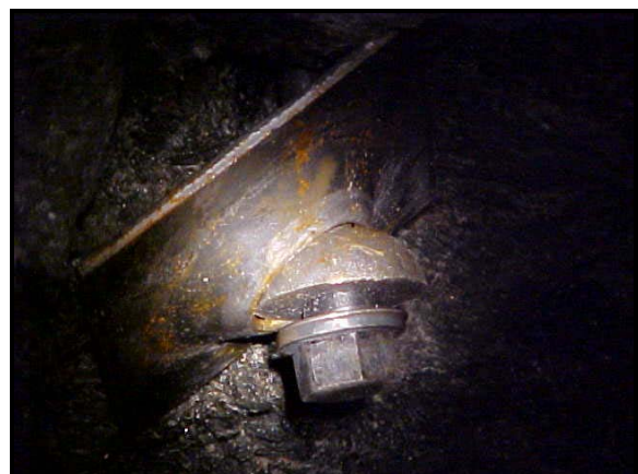
Forged-head support tendon showing load indicator that disappears when tensioned
