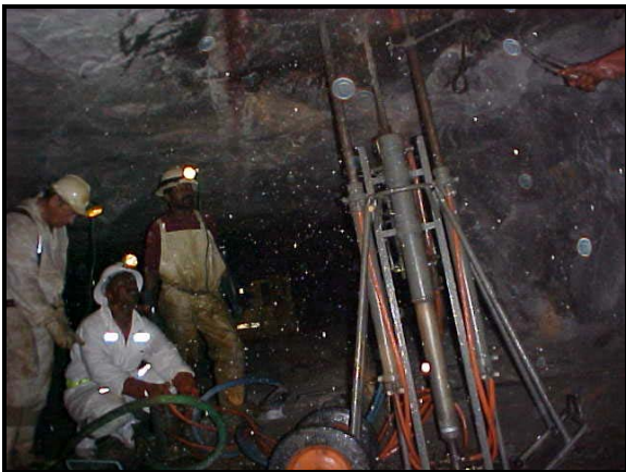
Small, portable roofbolt-drilling rig in action – note remote control operation
