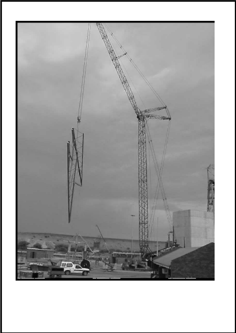
Figure 4 First pre-assembled section being lifted
