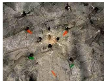
Figure 16. Photograph of spiral connection of a burn cut with Splitters
