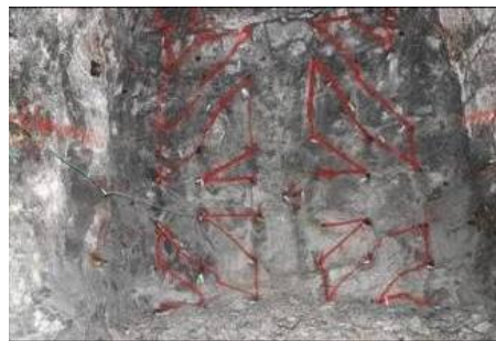
Figure 15. Photograph of Reef Master® connection in quarter spiral – chevron format
