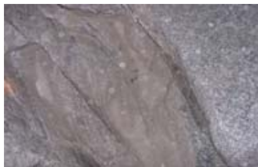
Figure 9 – showing lining eroded on lamprophyre dyke exposure
