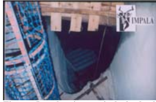
Figure 5 – showing typical ringback ladder installation
