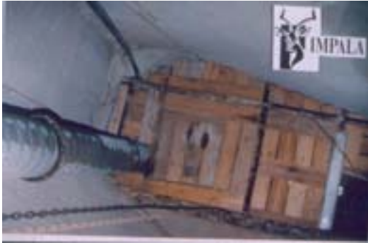
Figure 4 – showing typical working platform
