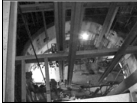
Figure 22: Main Shaft equipping
