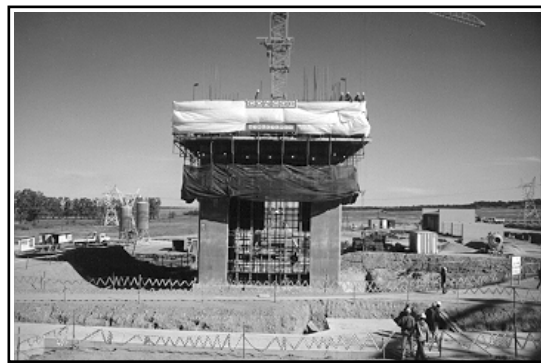
Figure 8: Main Shaft Slip Form
