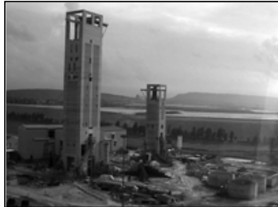
Figure 1: South Deep twin shafts
