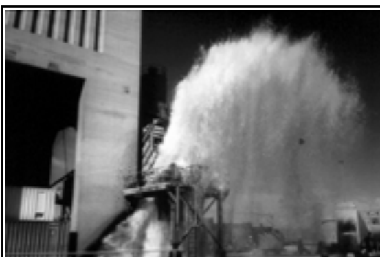
Figure 10: Baling water from the main shaft
