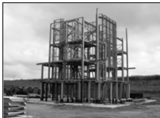
Figure 21: Station pre-assembled on surface
