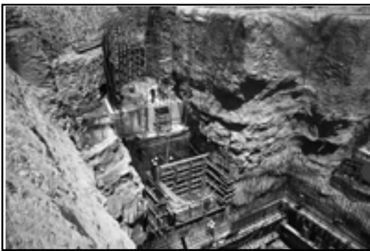
Figure 7: Main Shaft Headgear box cut
