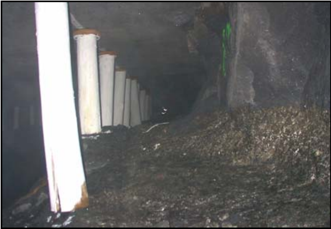
T/Cut after blast (2m shoulder)
