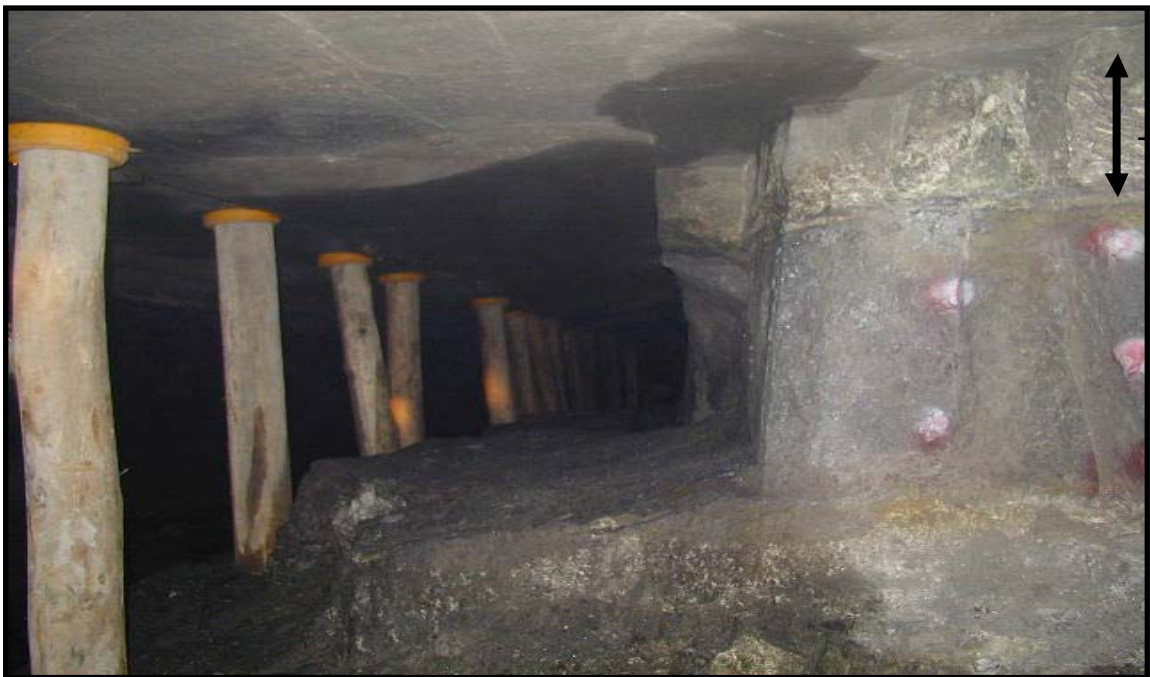
T/Cut showing the distinct waste porting between reef and hanging wall of 15 – 25cm
