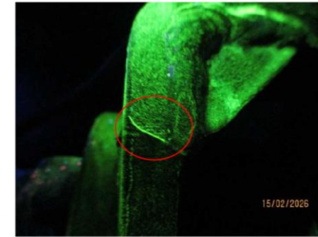
Fig 3: Chairlift No: SI/43 Crack like indications noted.
