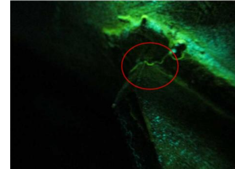
Fig 4: Chairlift No: Carrier SI/149 Crack like indications noted.
