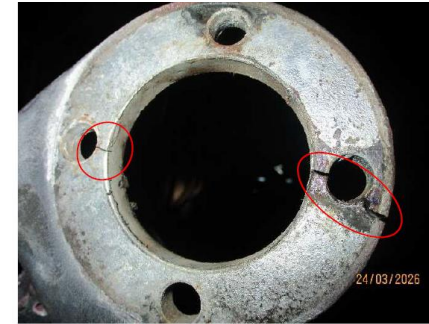
Fig 20: Chairlift No: SI/21 Crack like indications noted.
